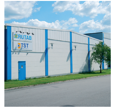
Warehouse - and production facility in Nässjö, Sweden
